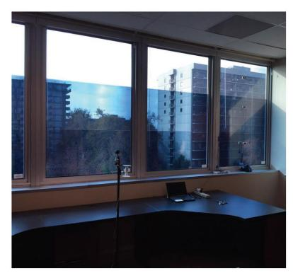
Figure 32: Each window pane had three sub-zones that could be independently controlled (Fernandes et al. 2018, p.14)
