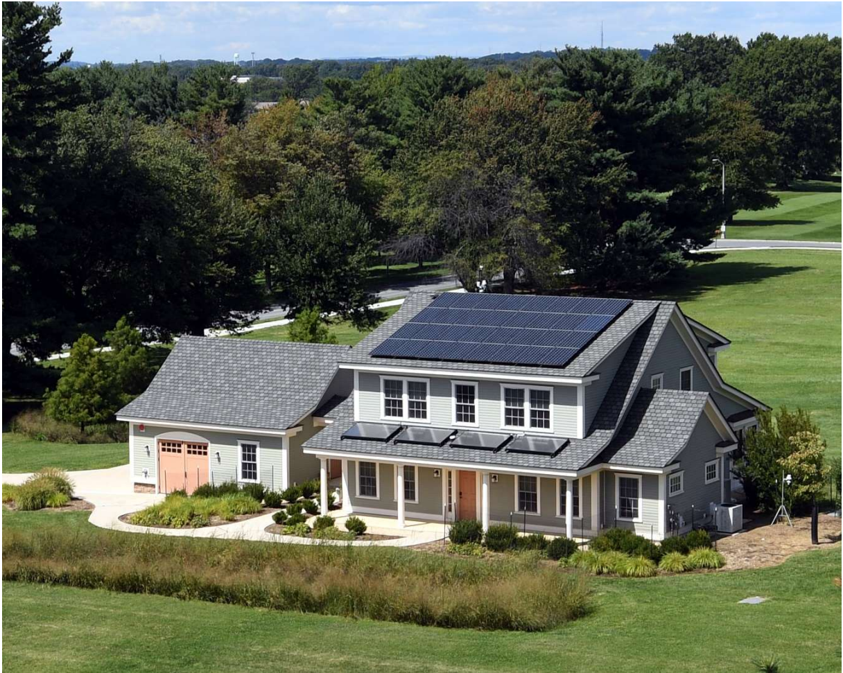
Figure 20: NZERTF south view
