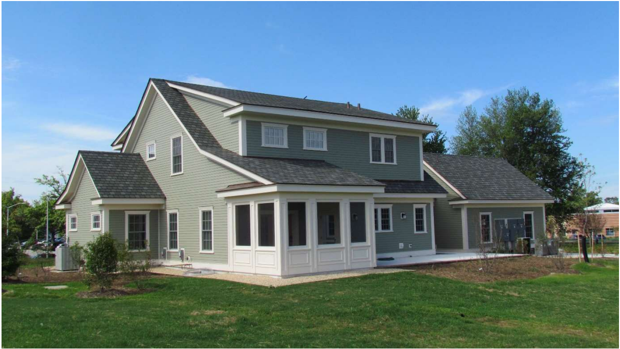
Figure 21: NZERTF north view
