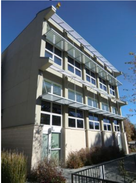
Figure 10: Shading system of the south facing facade of the Southface office building in Atlanta, GA, USA
