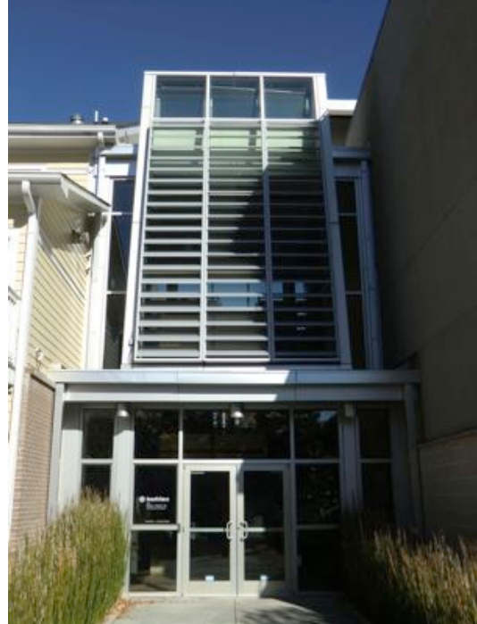
Figure 11: Shading system of the south facing entrance of the Southface office building in Atlanta, GA, USA
