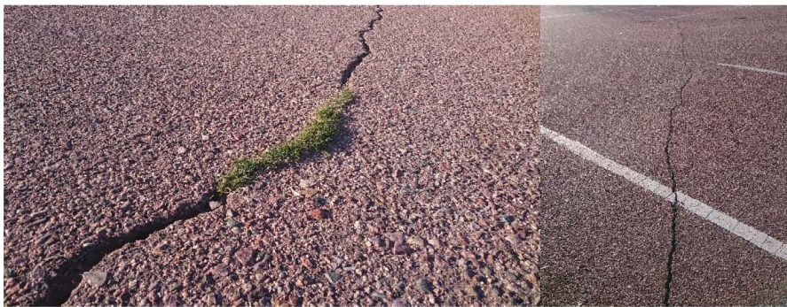
FIGURE 13 : Thermal Cracks in Roosevelt, Arizona
