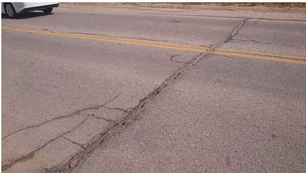
FIGURE 13 : Thermal Cracks in Roosevelt, Arizona
