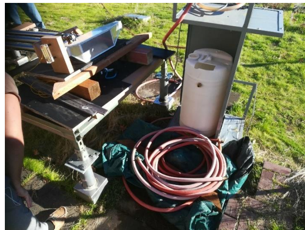
Figure 21. Emptied evacuated tubes, tank and the disconnected tubes.
