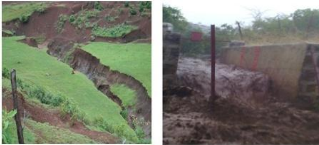
Figure 25 Gully development in the upper part of the watershed (left) runoff with high sediment concentration at the outlets (right)
