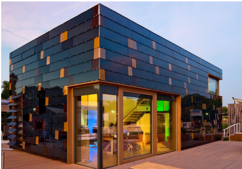
Figure 3: surPLUShome’s innovative solar panel façade. Source: https://www.solardecathlon.gov/past/2009/team_germany.html
