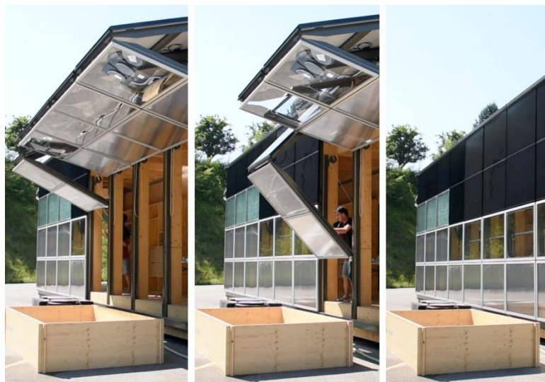
Figure 1: NeighborHub ‘Exterior Skin’ façade. Source: http://www.swiss-living-challenge.ch/en/swiss-living-challenge/
