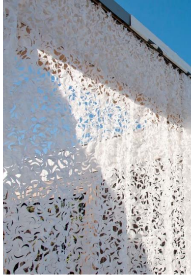
Figure 6: Detail of LISI house's façade. Source: Photo by Kirra McCollum
