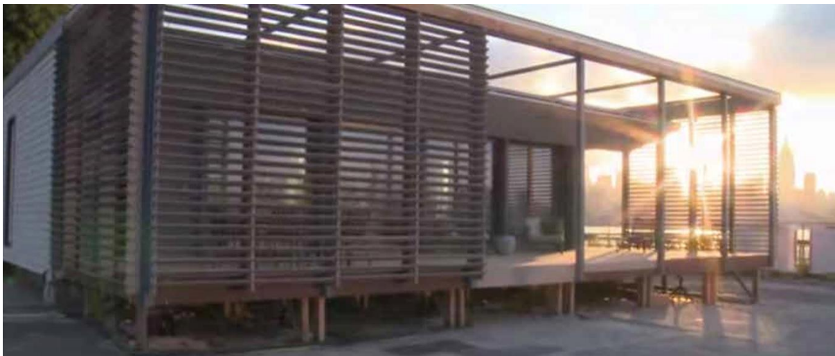
Figure 2: SURE house storm protecting façade. Source: https://www.solardecathlon.gov/2015/assets/pdfs/sd2015_narrative_sit.pdf
