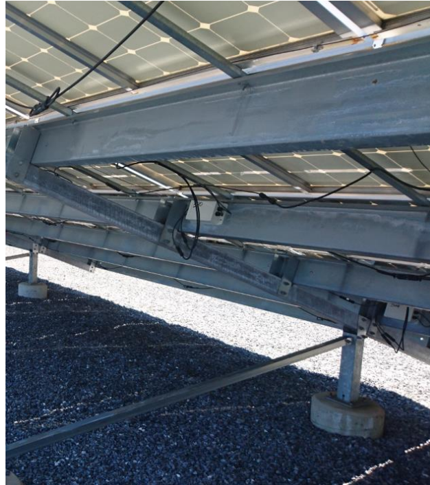
Figure 32 IV curve tracers on the mounting structure (own picture)
