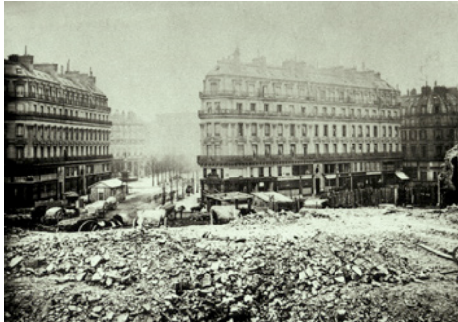
Fig. 15: Demolition of medieval districts in Paris around 1870.
