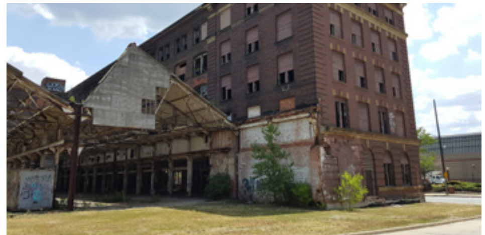
Fig. 56: The connection of the assembly hall to the main building.
