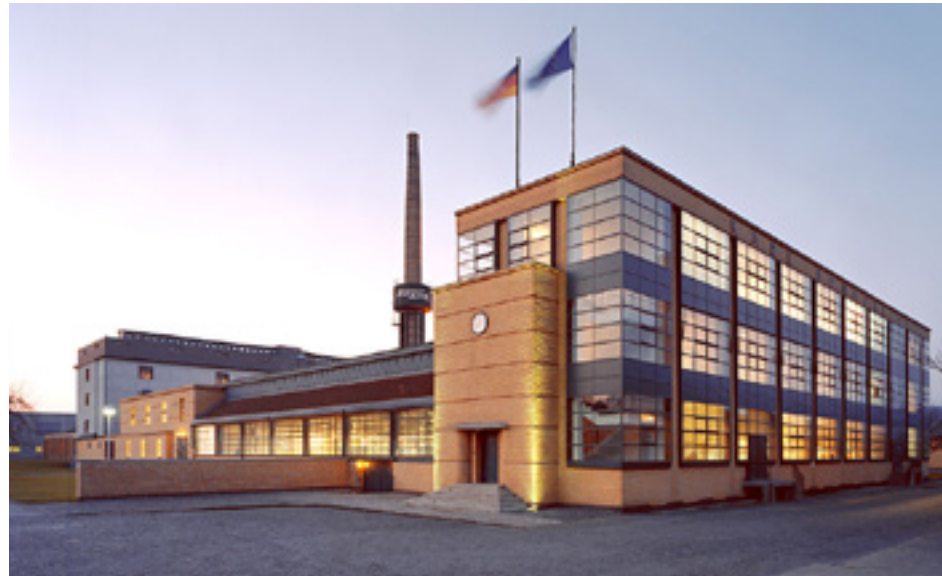
Fig. 21: The Fagus Factory by Walter Gropius and Adolf Meyer opened in 1913, being an early example of Modern architecture. The glass facade and especially the corner detail without a load bearing element were revolutionary.
