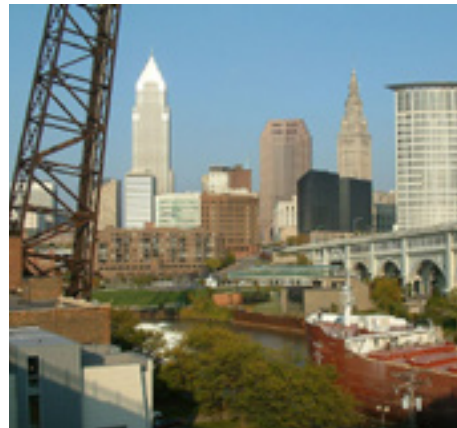
Fig. 13: Industrial buildings and infrastructure near downtown Cleveland.
