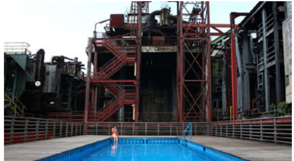
Fig. 17: Zeche Zollverein in Essen (Germany): successfully reusing the structure has converted the public opinion about it and turned it into an important cultural venue.
