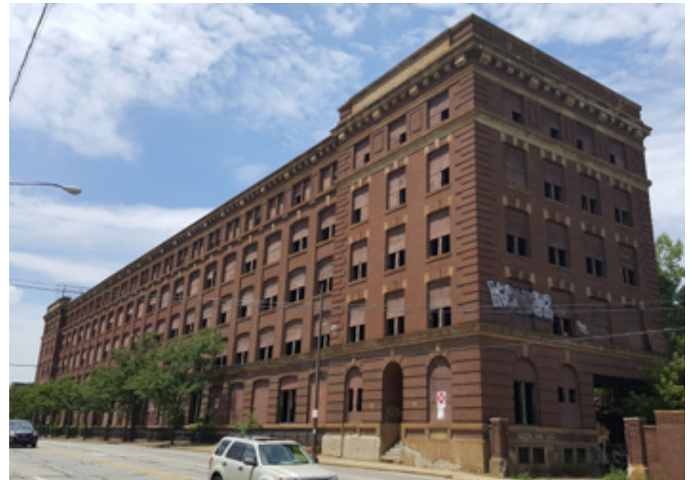
Fig. 44: The 122m long south facade of the main building of the Warner & Swasey Complex, facing Carnegie Avenue.
