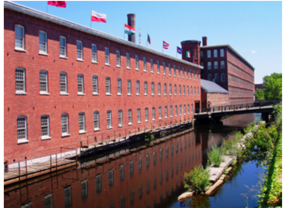
Fig. 38: The complex is surrounded by canals that were needed to create the waterpower in the early days of the mills.
