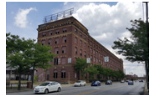
Fig. 47: The Warner & Swasey Building
