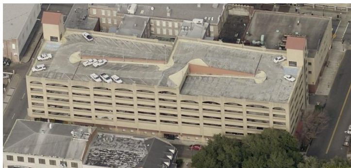
Figure 31: Aerial photography - State Street Garage [SAGIS, 2015]
