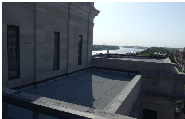
Figure 38: City Hall roof [Wimmer, 2015]
