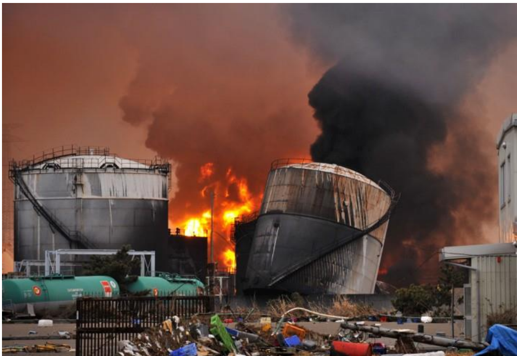
Figure 4 – burning petroleum refining plant in Shiogram/Japan, after an earthquake and tsunami 03/13/2011 9
