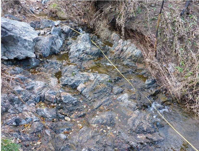
Figure 3: An example of complex jointing that was deemed too difficult to accurately identify and measure. Note tape measure for scale.
