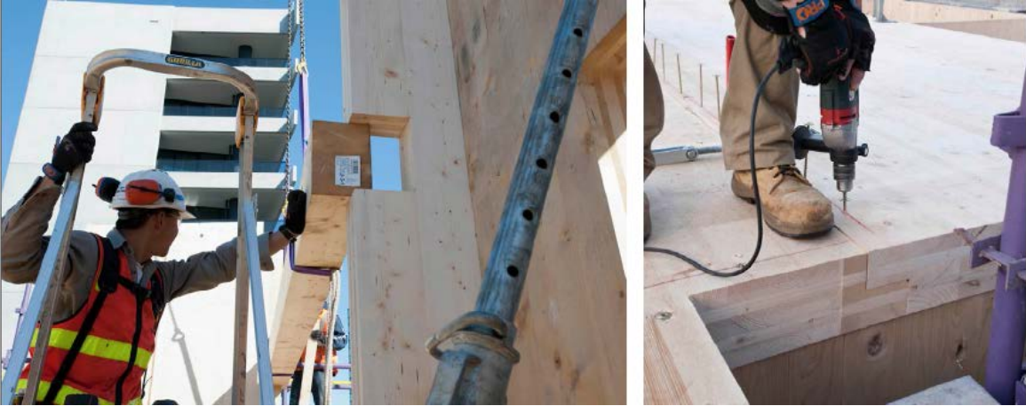
Figure 19: Construction work 'Forté' (Lend Lease, 2013). Courtesy of Lend Lease
