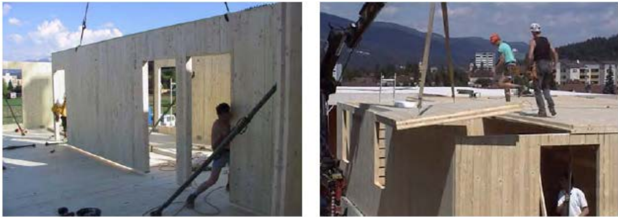
Figure 9: Images of platform construction (Augustin, 2008). Courtesy of Institute of Timber Engineering and Wood Technology, TU Graz
