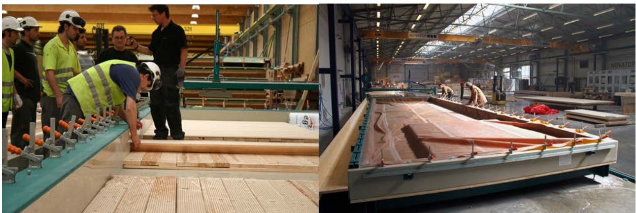
Figure 30: CLT layup in vacuum press (right) sealing with vacuum sheet (right). Courtesy of Woodtec Fankhauser
