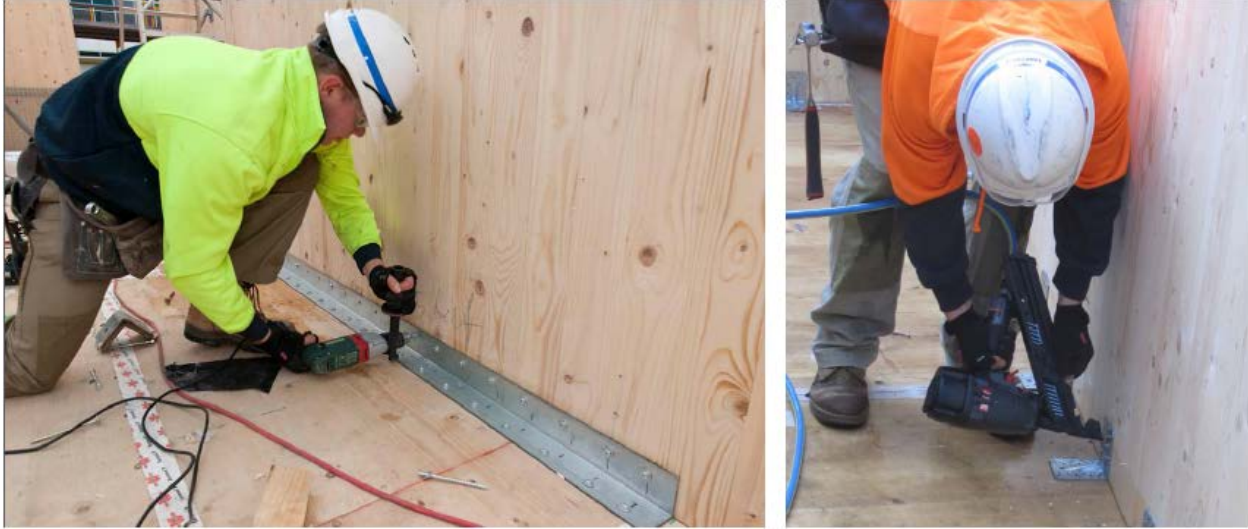
Figure 20: Construction work 'Forté' (Lend Lease, 2013). Courtesy of Lend Lease
