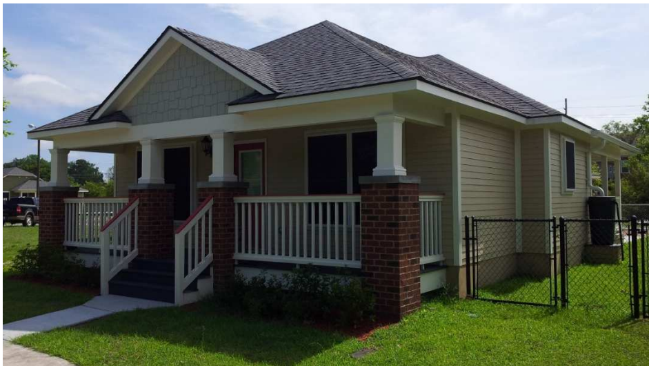
Figure 42: Image - "12 Greencottage Way" Front View [Source: own Figure]
