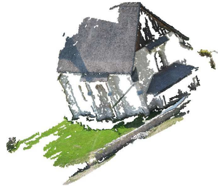
Figure 20: 3D Reconstruction of Old Church from Visual-SFM
