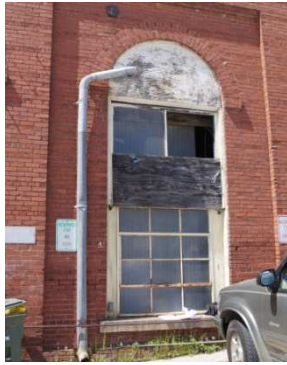
Figure 28: On-site visit, windows 1
