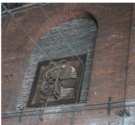
Figure 31: On-site visit, closed openings 1
