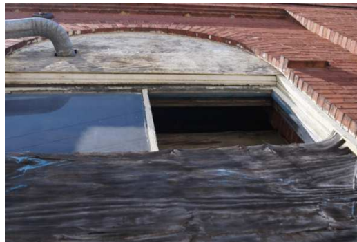
Figure 30: On-site visit, windows 3
