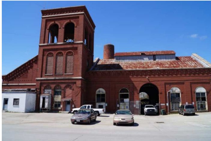
Figure 25: On-site visit front entrance
