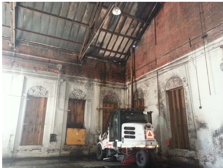
Figure 34: On-site visit, Interior Stucco [P Felder & Associates, 2014]
