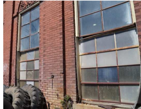
Figure 29: On-site visit, windows 2
