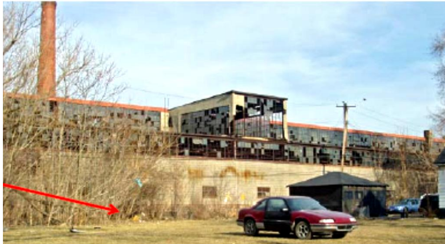
Figure 13 Illegal parking, vacant lots with cars Unpaved and no parking stripes Photographed by Andrea Korber 2014
