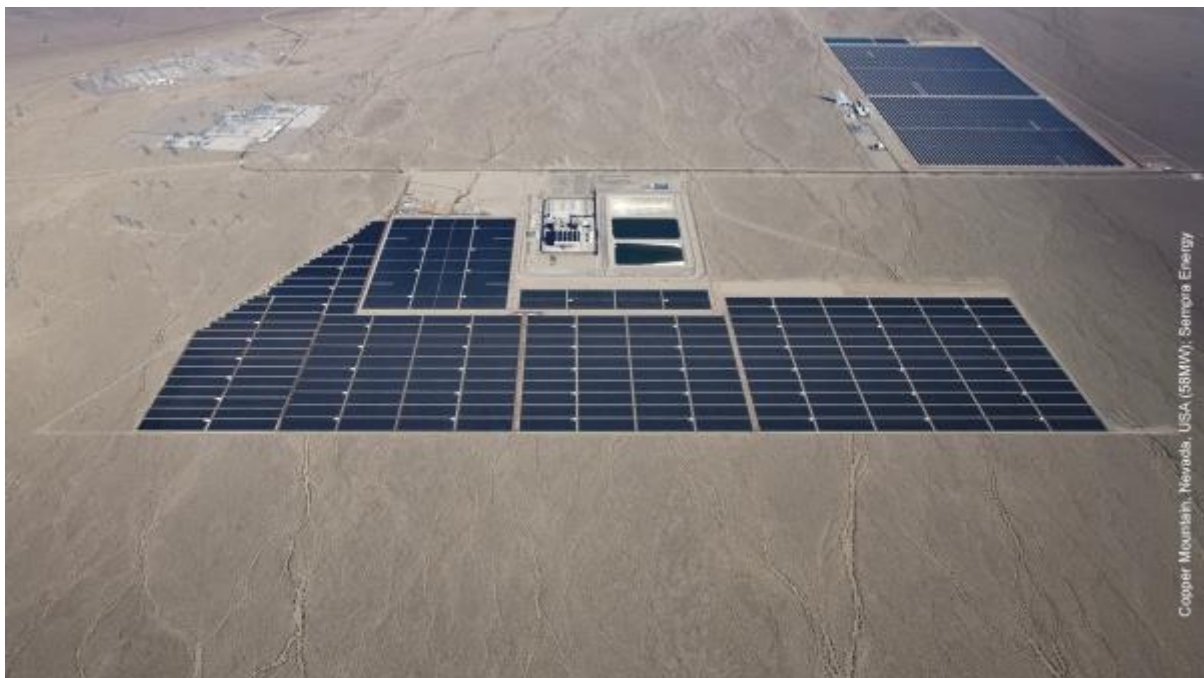
Figure 28: Copper Mountain Solar 1 [cf. 29]
