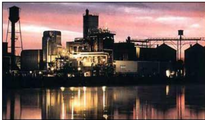
Figure 30: Agrilectric power partners facility [cf. 31]
