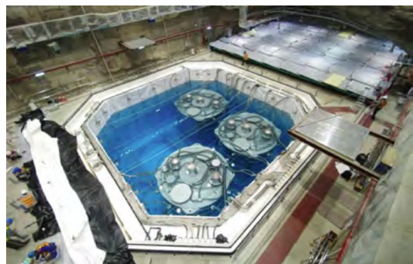
Figure 11: Water pool during construction
