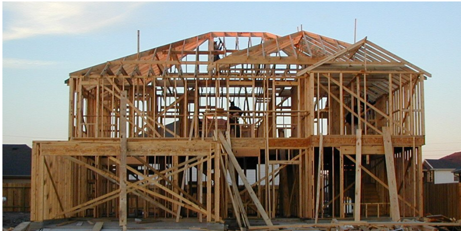
Figure 4. Typical wood framed home (photo from brijetblog.com)
