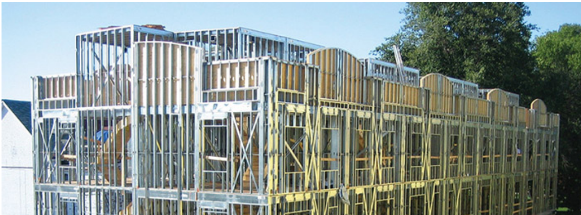
Figure 5. Typical light steel framed building (photo from urbannirmaan.com )
