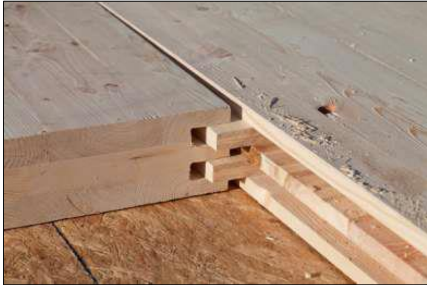
Figure 6: Double internal spline for panel connections
