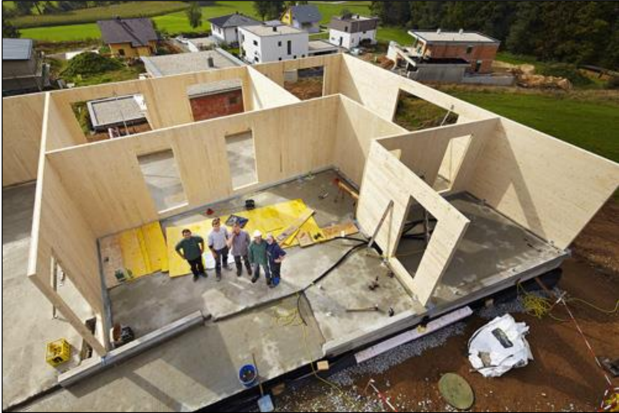
Figure 7: CLT construction example
