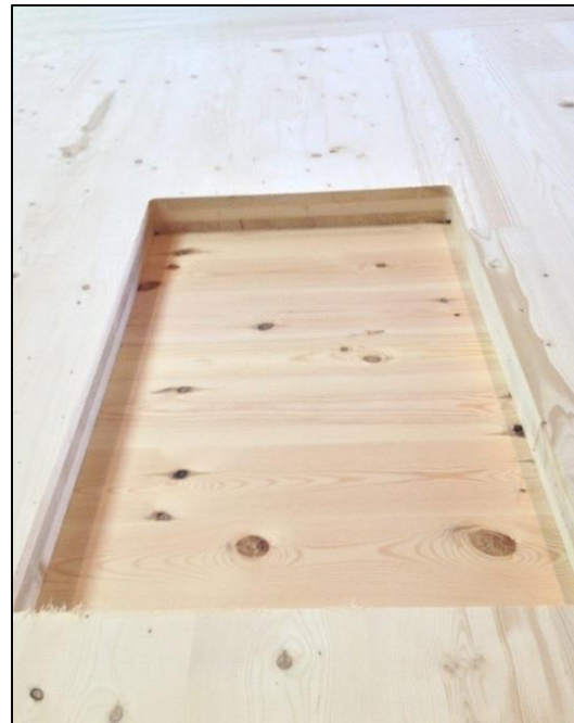
Figure 5: Finished CLT panel with CNC cutout likely for window installation (Stauder 2013)
