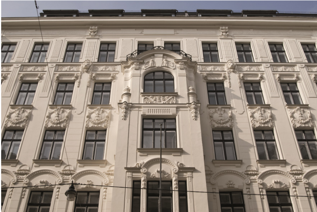
Fig. 1: Front of a wilhelminian building
