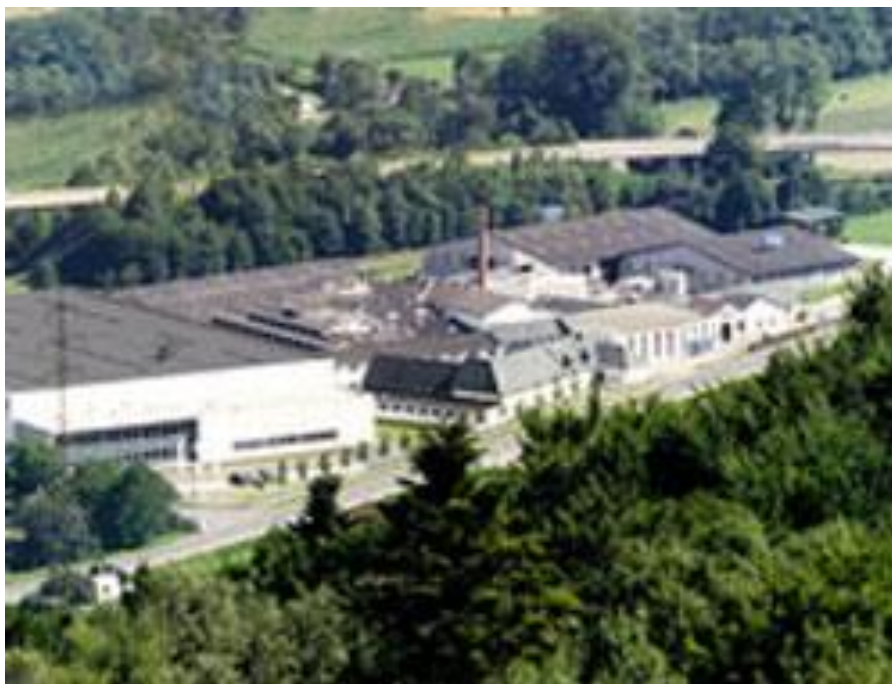
Figure 1: Plant in Grimmenstein
