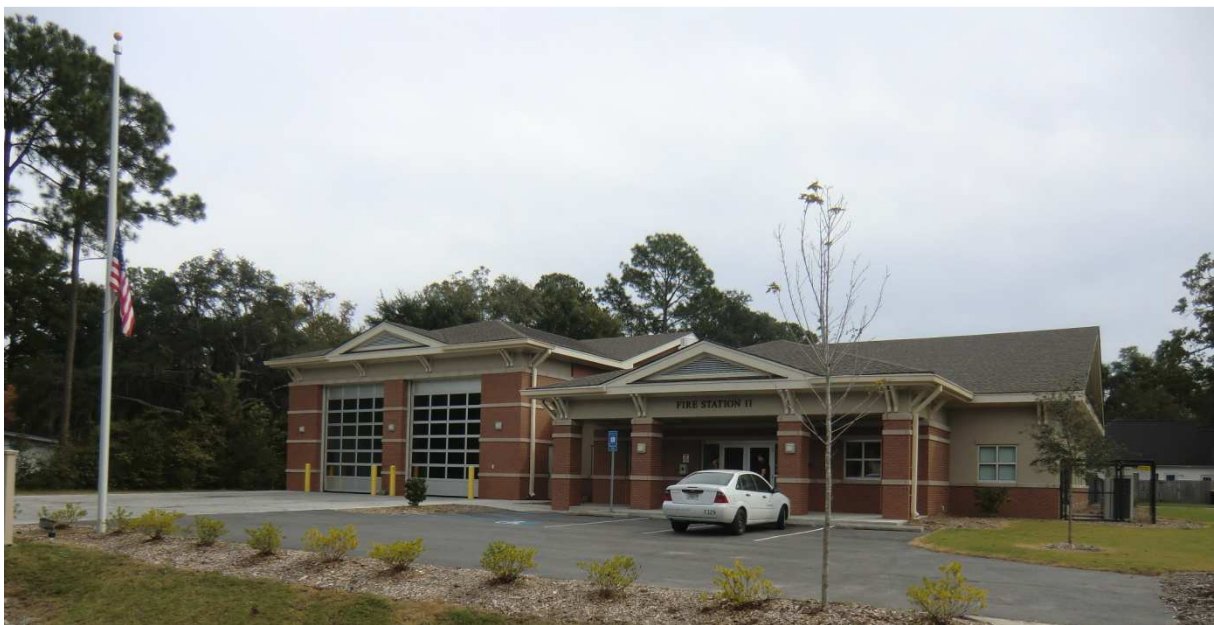
Figure 36: Fire Station 11, Savannah, 19.10.2012
