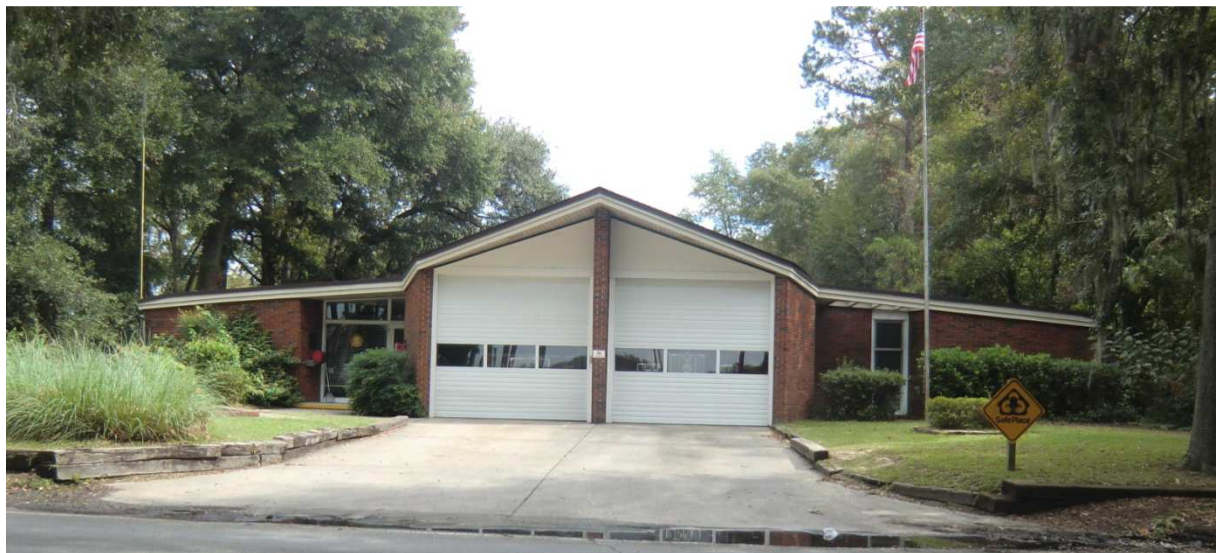
Figure 31: Fire Station 8, Savannah, 19.10.2012
