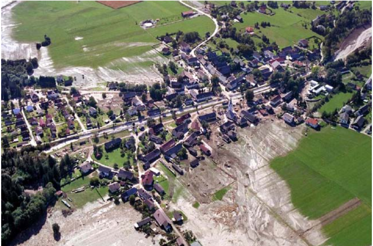
Figure 1-3: The village of Vorderberg after the inundation in 2003 (ROHNER et al., 2004)
