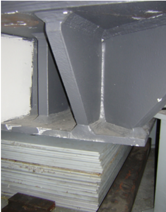
Fig. 64: Steel plates adjusting surface settlements.
