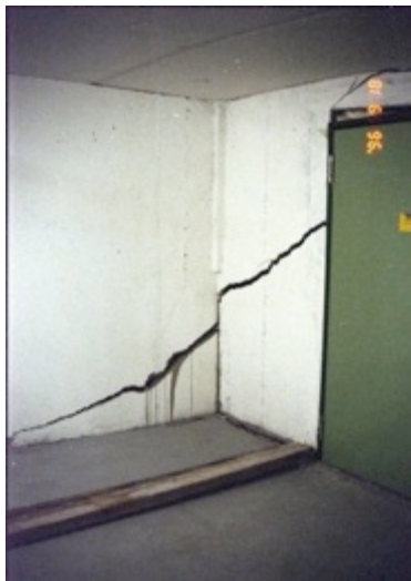
Fig. 59 + 60: Damages on Building (open Cracks and Deformation of roof).
