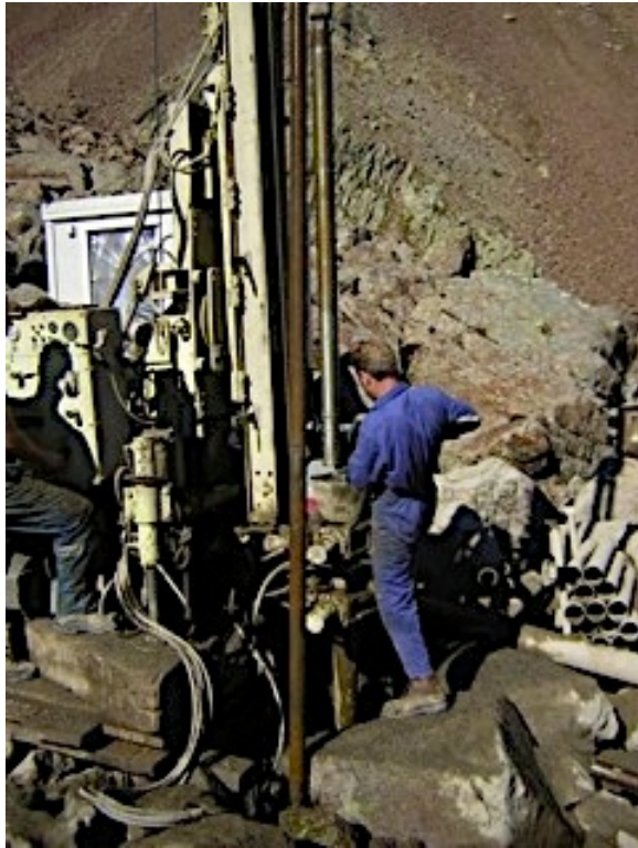
Fig. 71: Casing the borehole.
