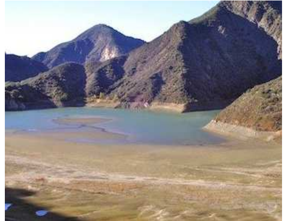
Fig. 2. Siltation of a hydropower reservoir (China)
