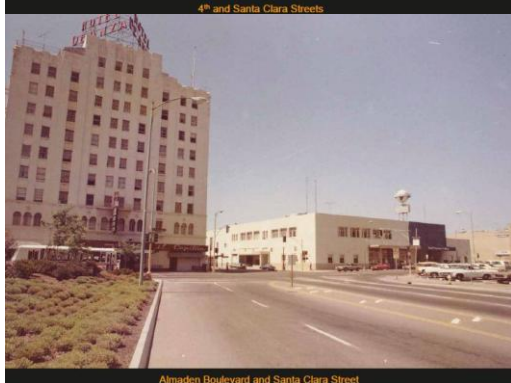
Almaden Boulevard and Santa Clara Street
