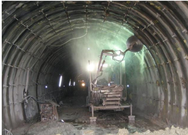
Figure 9, Execute saw cut (source Beton- und Monierbau)
