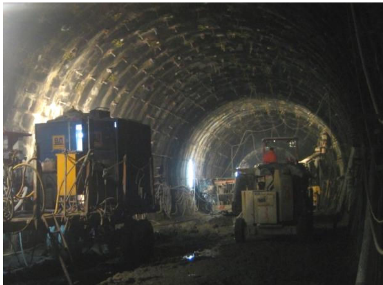
Figure 22, grouting process (source Beton- und Monierbau)
