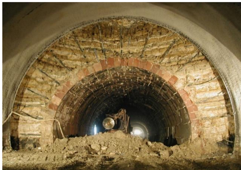
Figure 27, tunnel enlargement – Phase 2, photography (source Beton- und Monierbau 2007)
