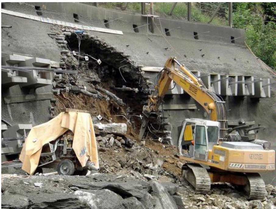
Figure 23: Excavation beneath a pipe umbrella 94
