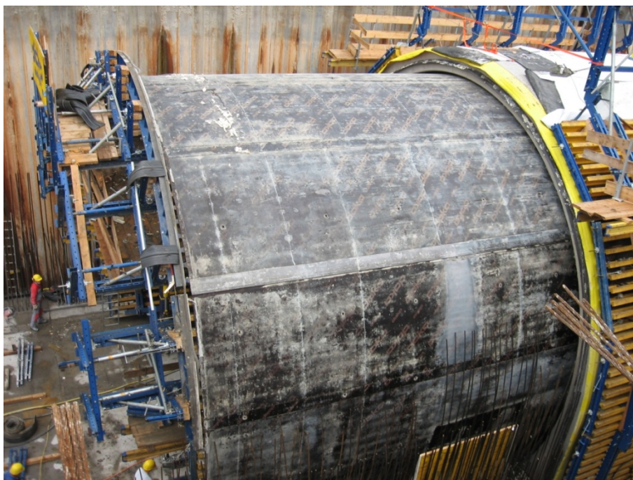
Figure 3: Use of Bottom Up at the Brenner railroad track
