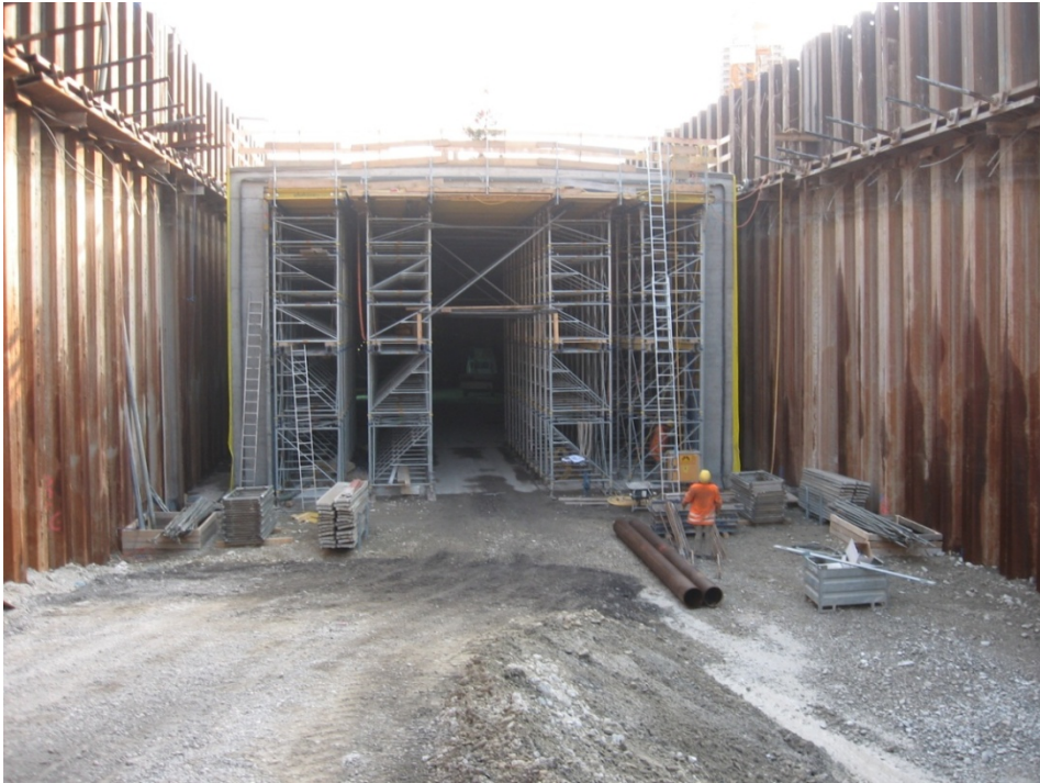
Figure 5: Use of Bottom Up at the Brenner railroad track
