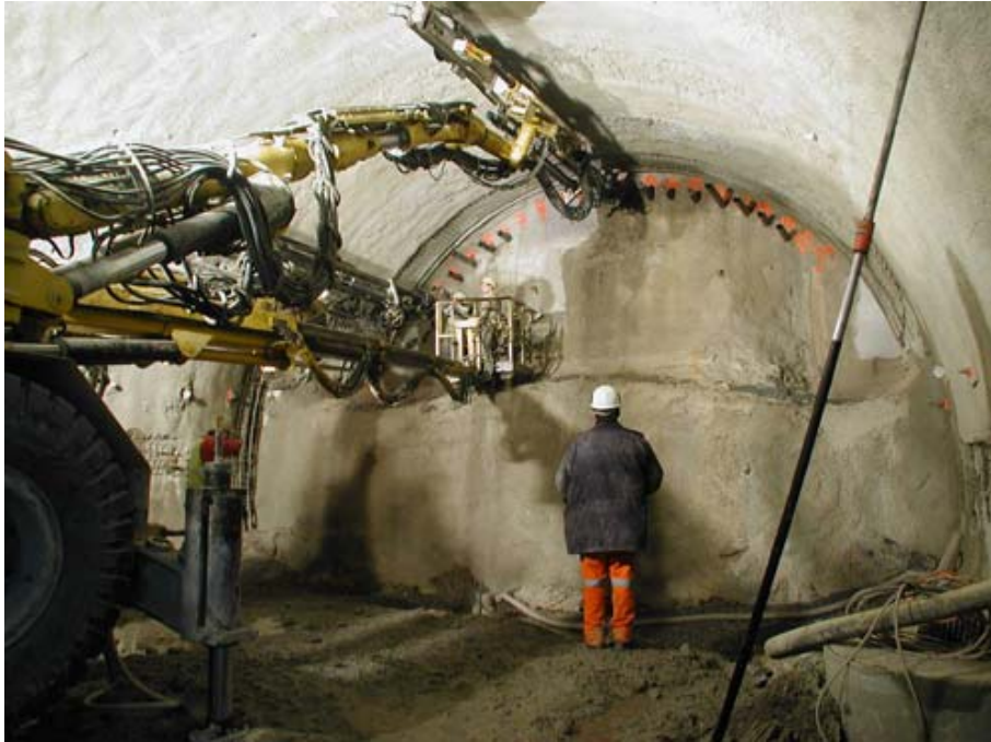
Figure 22: Installation of a pipe umbrella 93
