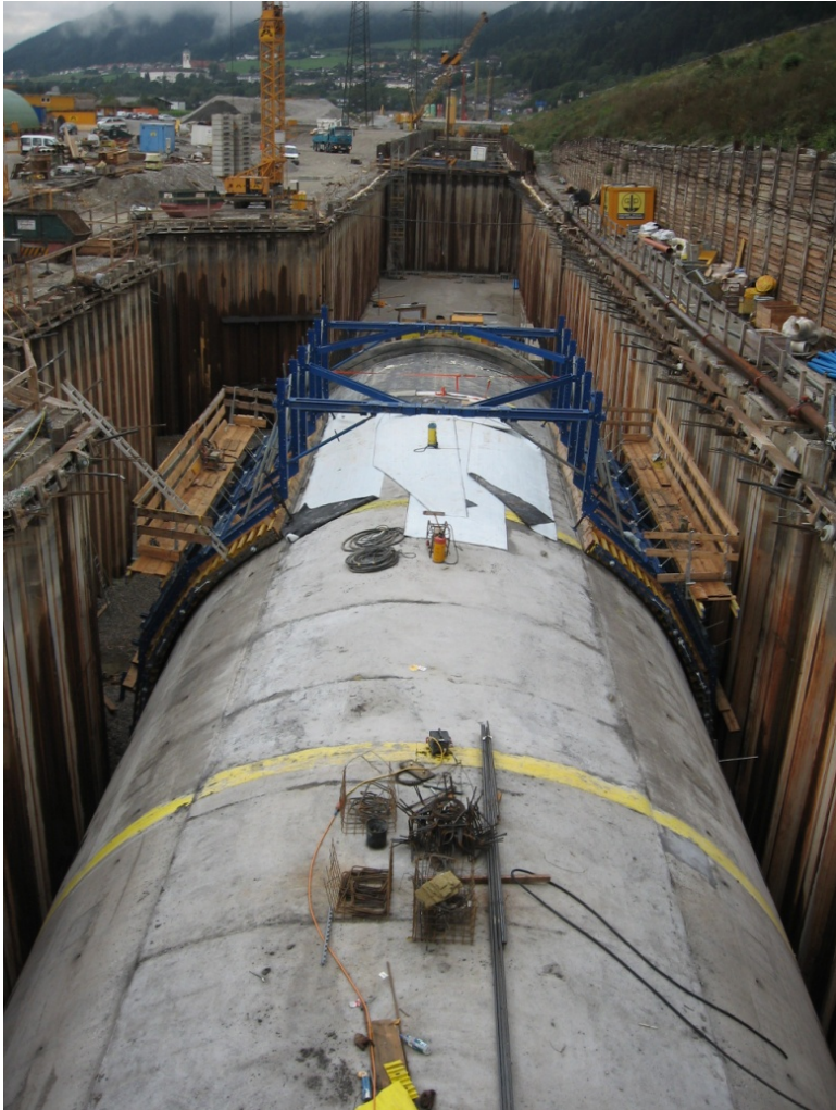
Figure 4: Use of Bottom Up at the Brenner railroad track
